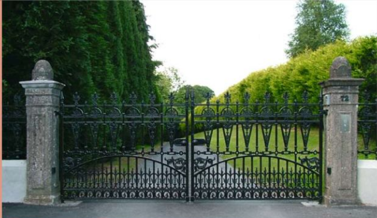
Gilberton driveway gates (12ft) hanging from existing stone gate pillars
