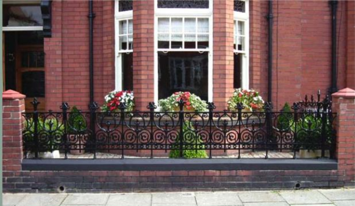
Prospect railings with posts
